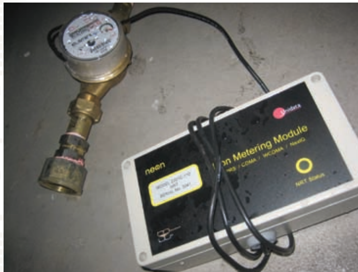
Figure 1 – Typical Meter and Logger Used for Flow Data Capture.
